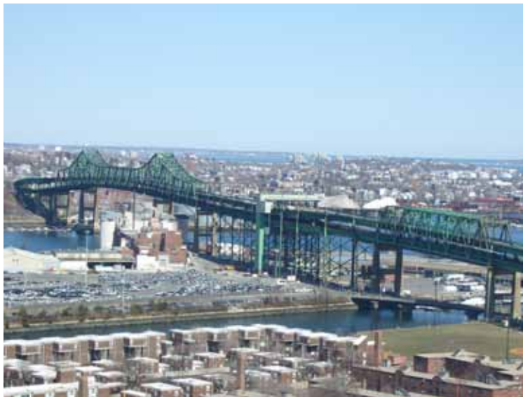
All-electronic tolling has begun on the Tobin Bridge and could soon come to the Massachusetts Turnpike.
